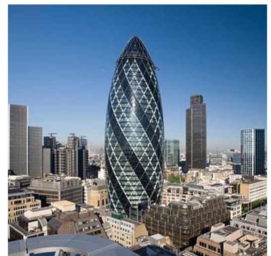
Figure 7: Gherkin, London, Designed by Foster + Partners
